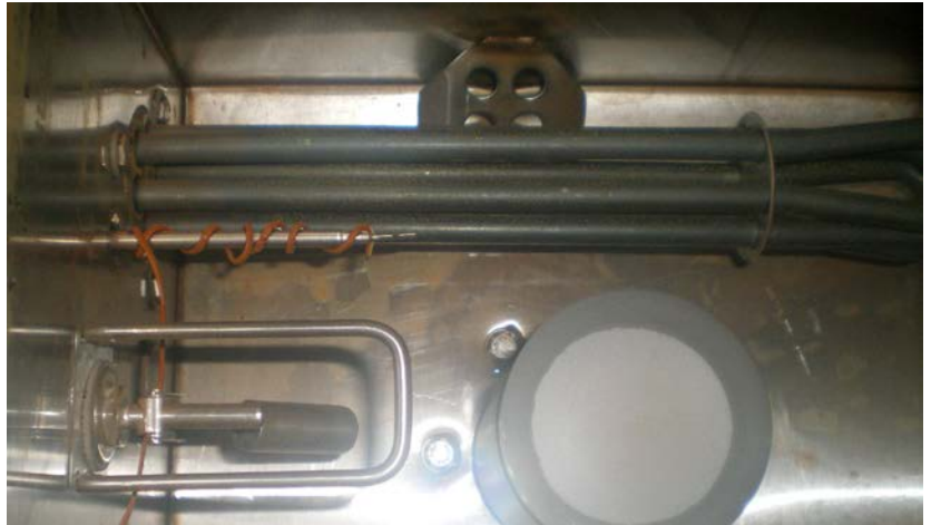
Figure 5: CMA-180 Tank Thermocouple location relative to factory temperature probe
