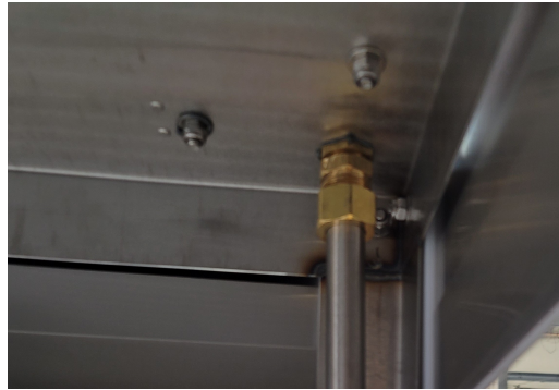
Compression fitting with stainless steel tube
